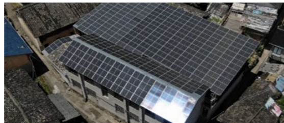
Roofing photovoltaic project
