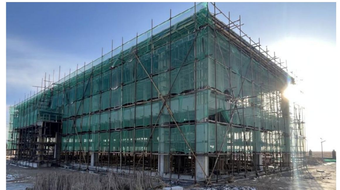
Construction site of "Mongolian Medical Hospital" of Sunite Right Banner
